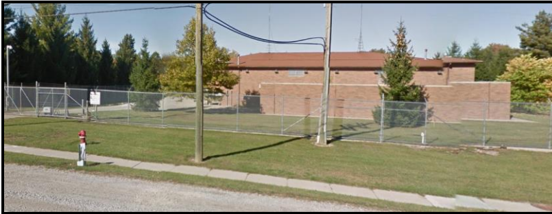
Figure V-29. Rochester Pump Station
