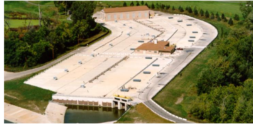
Figure V-38. Hubbell-Southfield CSO RTB
