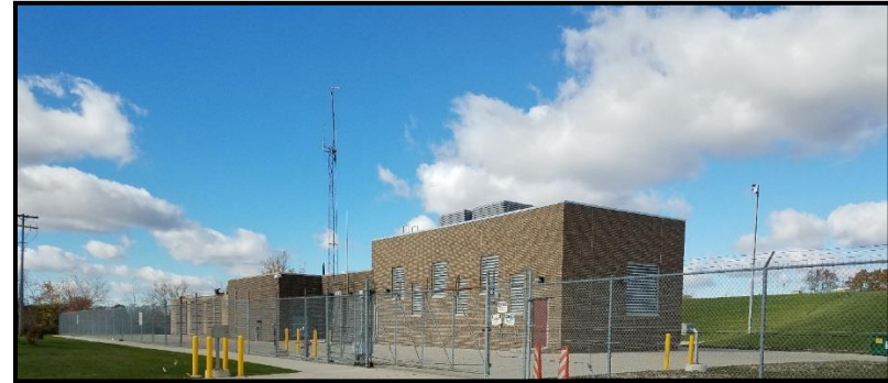
Figure V-33. Wick Road Pump Station
