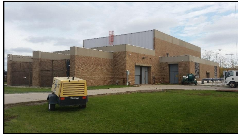
Figure V-55. Northeast Pump Station
