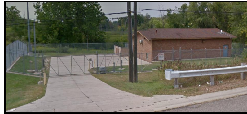
Figure V-28. Orion Pump Station
