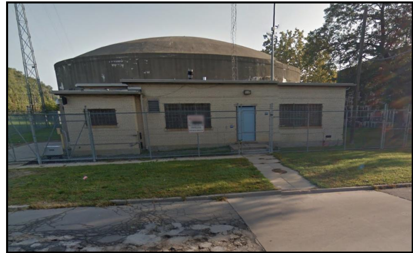
Figure V-18. Electric Avenue Pump Station
