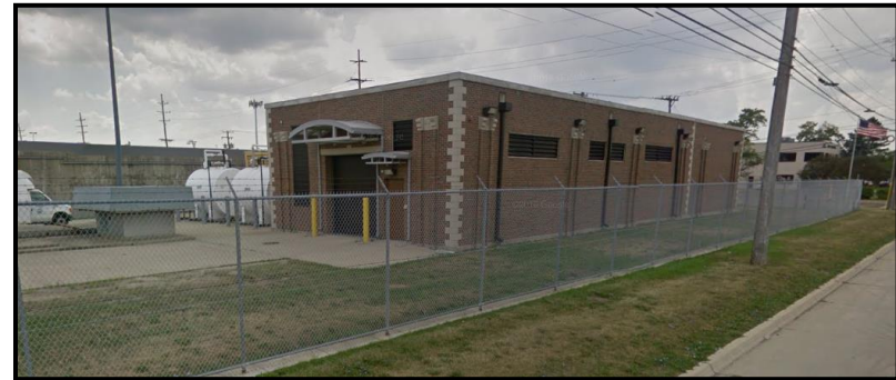
Figure V-31. Schoolcraft Pump Station
