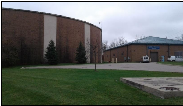
Figure V-19. Haggerty Pump Station
