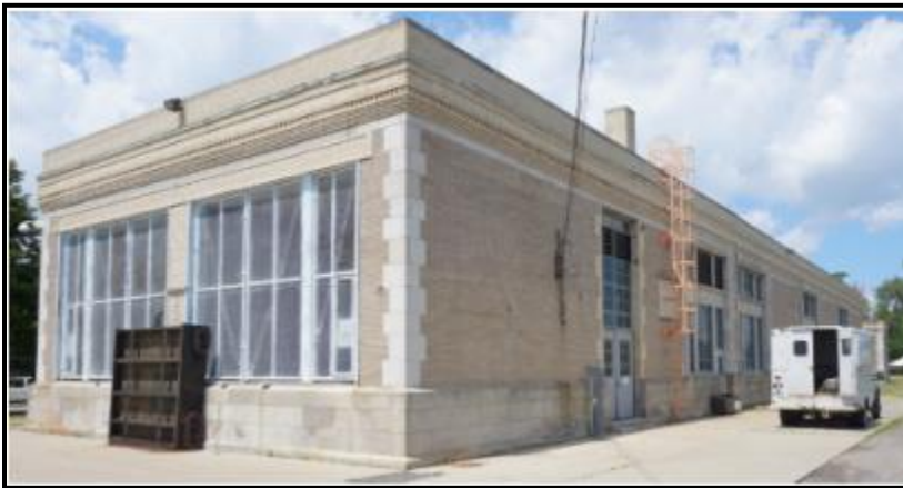
Figure V-51. Fairview Pump Station
