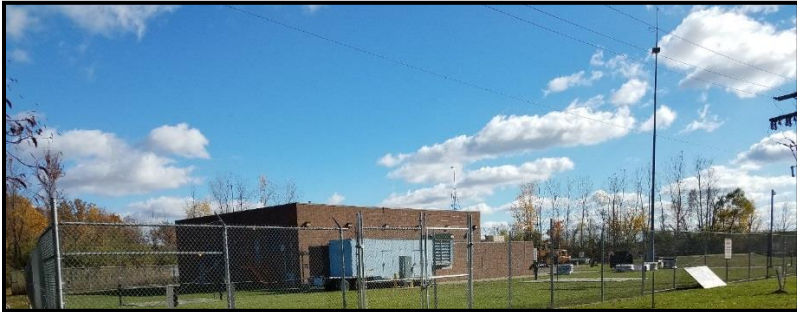
Figure V-34. Ypsilanti Pump Station
