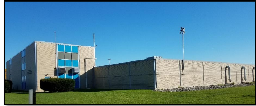
Figure V-20. Ford Road Pump Station
