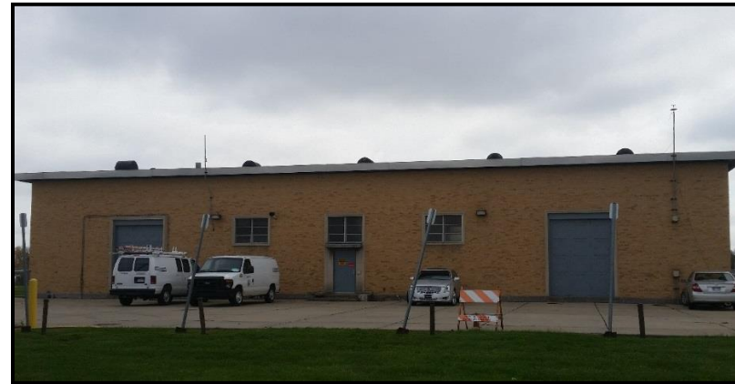
Figure V-26. Northwest Pump Station
