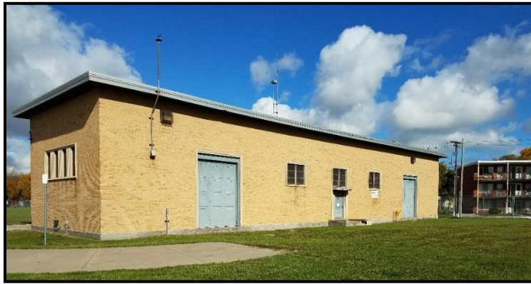
Figure V-17. Eastside Pump Station
