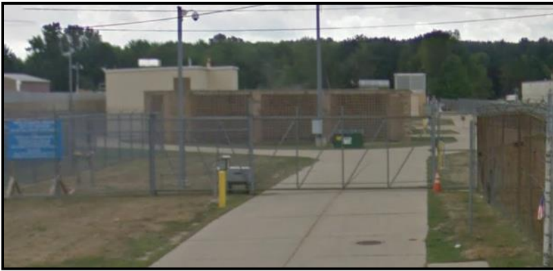
Figure V-23. Joy Road Pump Station
