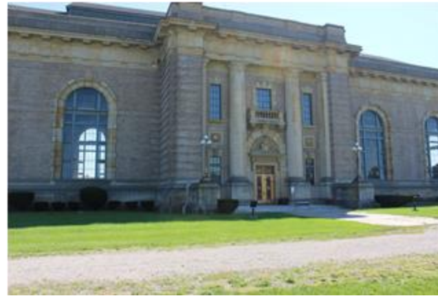
Figure V-10. Water Works Park WTP
