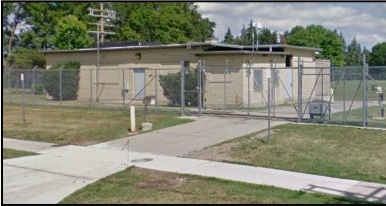
Figure V-32. West Chicago Pump Station
