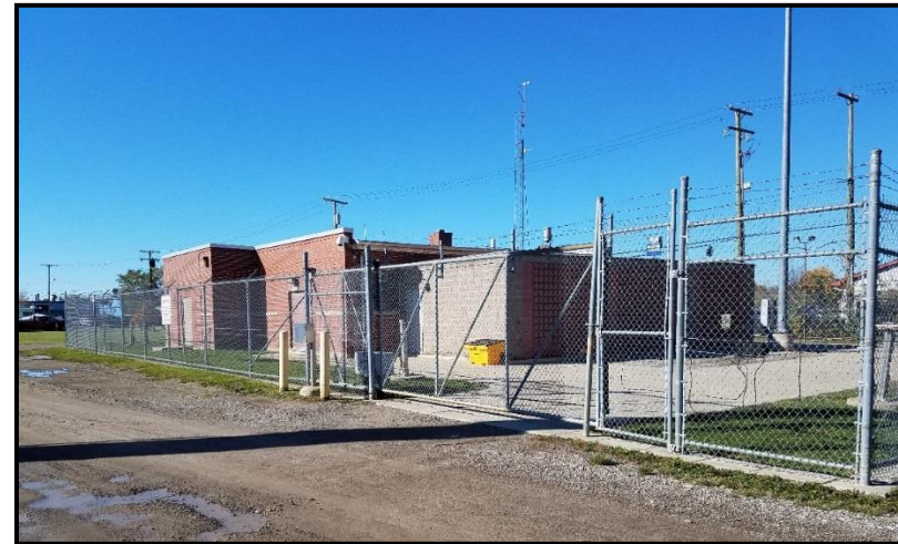
Figure V-22. Michigan Avenue Pump Station
