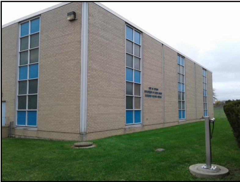
Figure V-25. Newburgh Pump Station
