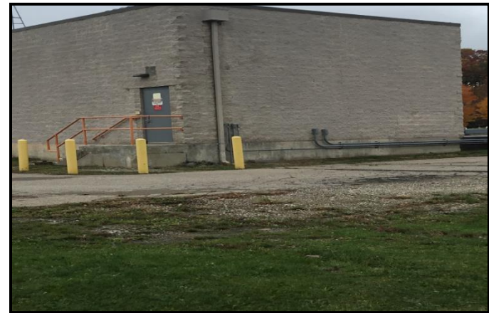
Figure V-16. Adams Road Pump Station
