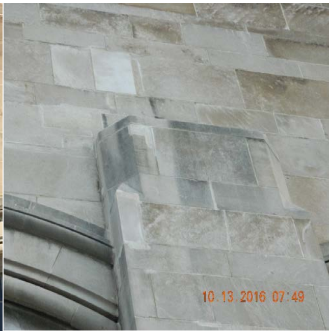
SPW High Lift Building – After
