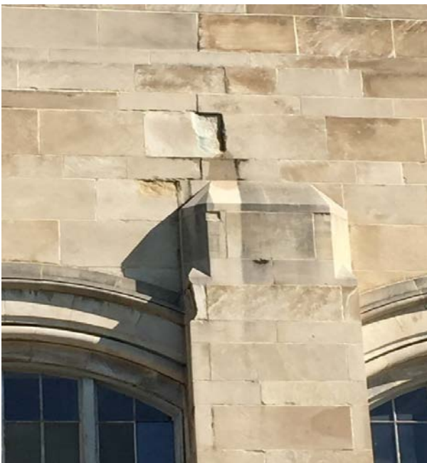
SPW High Lift Building – Before
