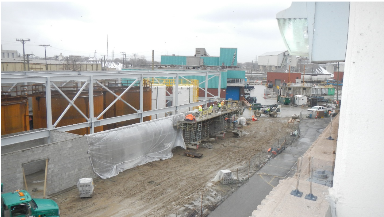
Hypo Building Construction
