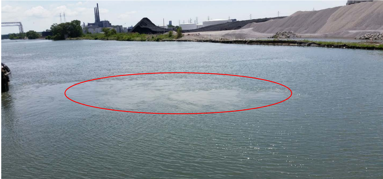
42-inch Water Main Break under Rouge River near WWTP on July 20, 2016
