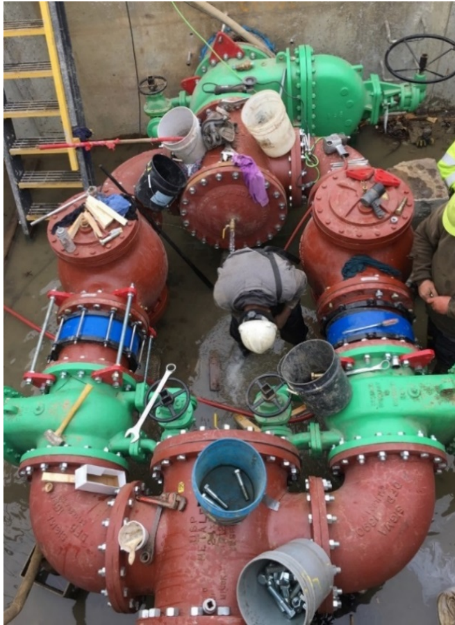
PRV Replacement Complete
