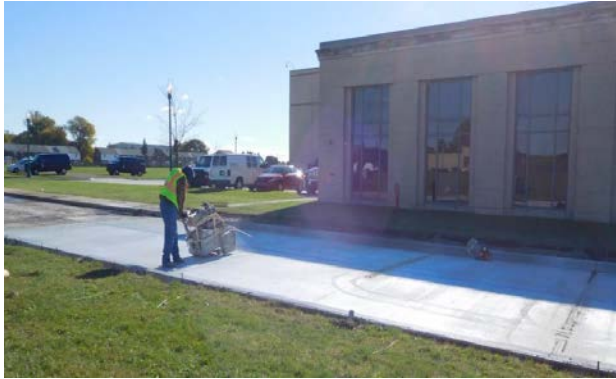
Administration Drive after repairs
