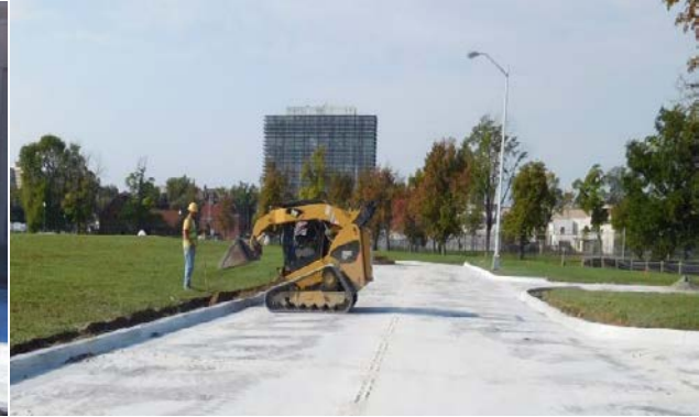
Restoration of H Drive
