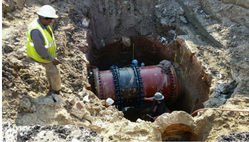
66-inch Straight Pipe Installed (after)
