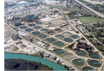
Aerial view of the WRRF
