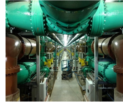
SP-563 – Rehabilitated 1958 Pipe Gallery (in progress)
