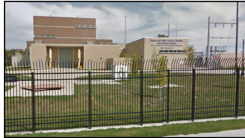
Figure VI-62. Oakwood Pump Station
