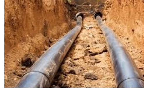
Water main installation
