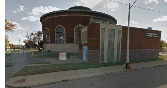
Freud Pump Station
