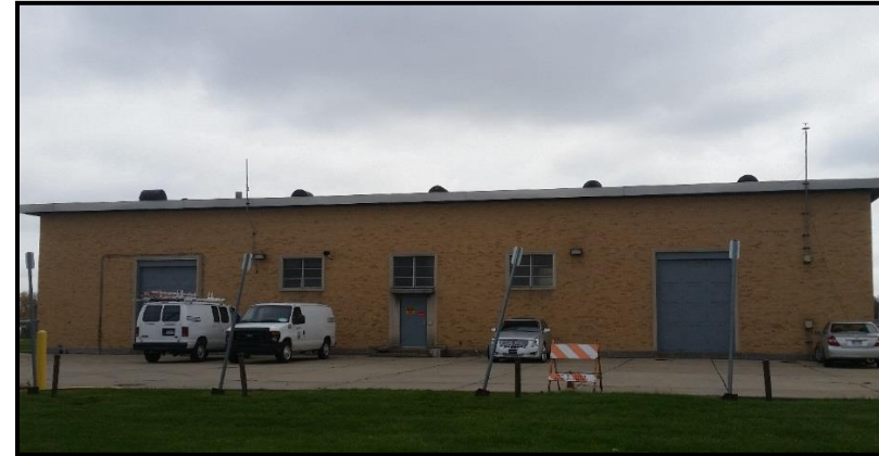
Figure VI-30. Northwest Pump Station
