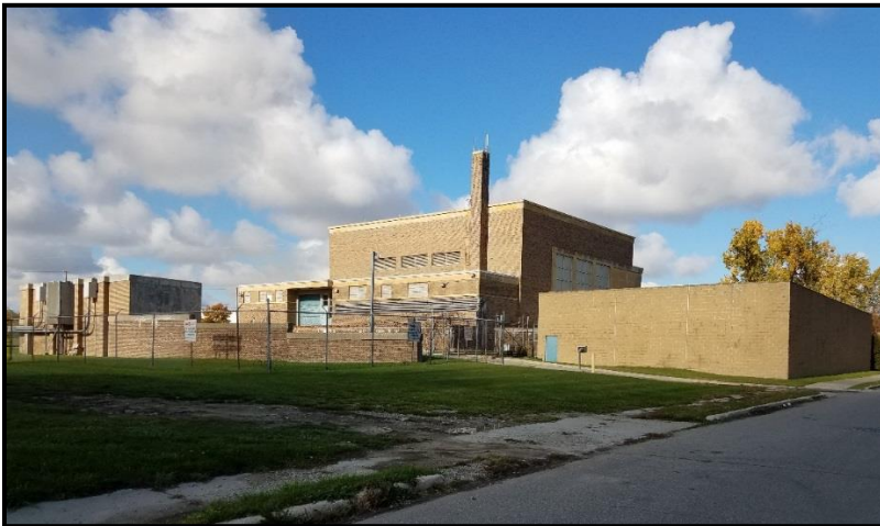
Figure VI-59. Freud Pump Station
