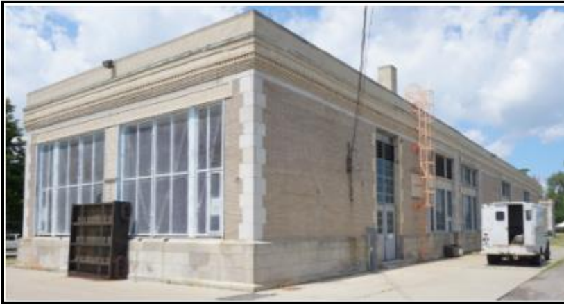
Figure VI-57. Fairview Pump Station
