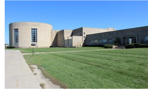
Northeast Water Treatment Plant
