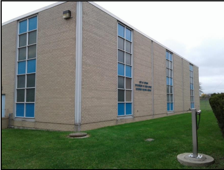
Figure VI-29. Newburgh Pump Station
