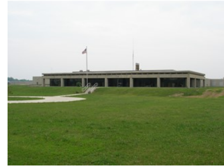
Lake Huron Water Treatment Plant
