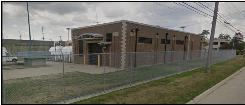
Figure VI-35. Schoolcraft Pump Station
