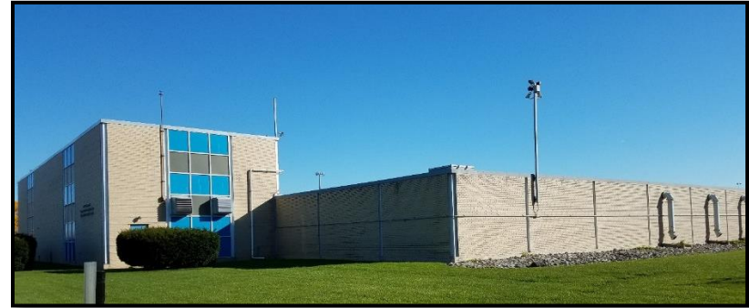
Figure VI-24. Ford Road Pump Station
