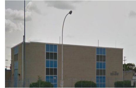
Ford Road Booster Pumping Station
