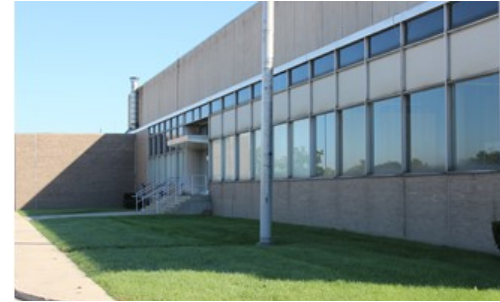
Southwest Water Treatment Plant
