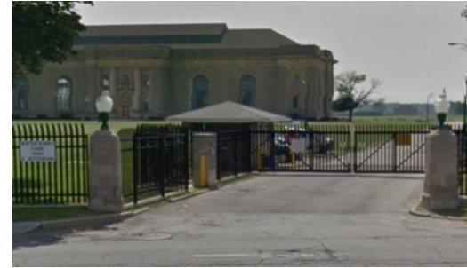
Waterworks Park WTP
