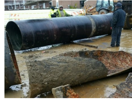
Water main replacement
