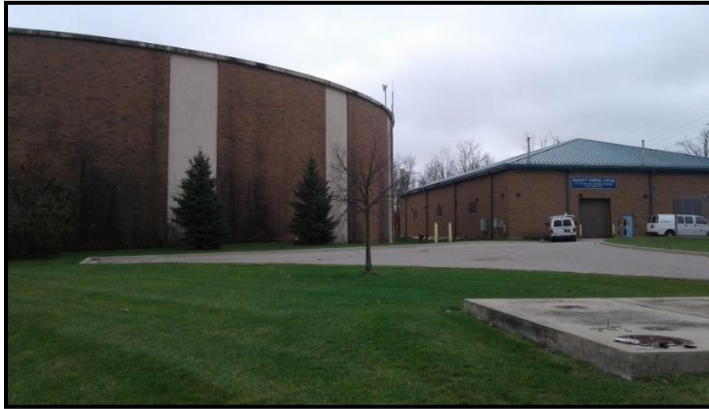
Figure VI-23. Haggerty Pump Station
