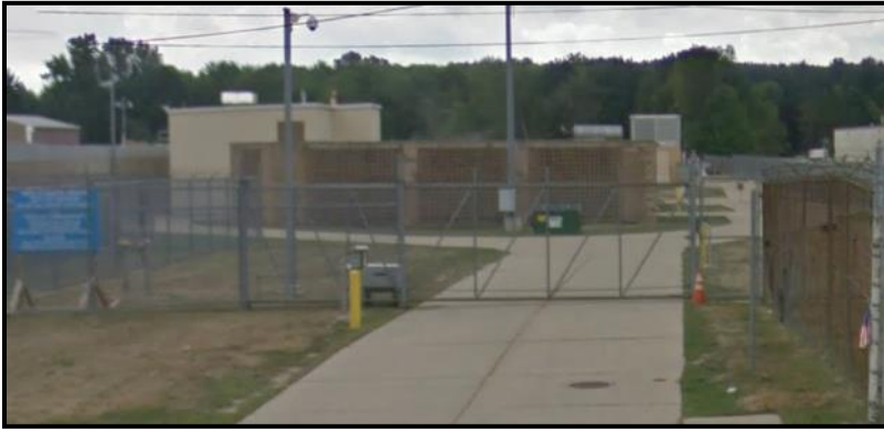
Figure VI-27. Joy Road Pump Station
