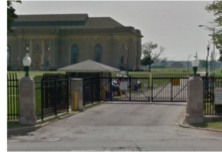
Waterworks Park WTP
