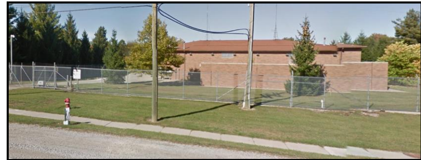
Figure VI-33. Rochester Pump Station
