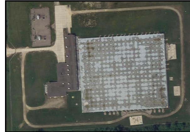
Figure VI-28. Imlay Pump Station
