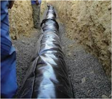
Water main being laid
