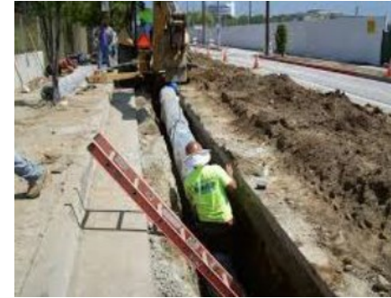
Water main being replaced
