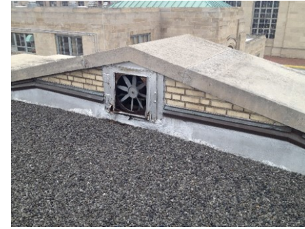
Filter Building roof
