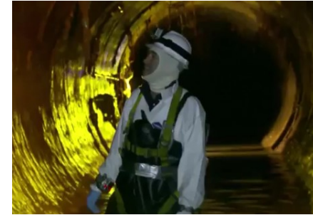
Visual inspection of a large sewer
