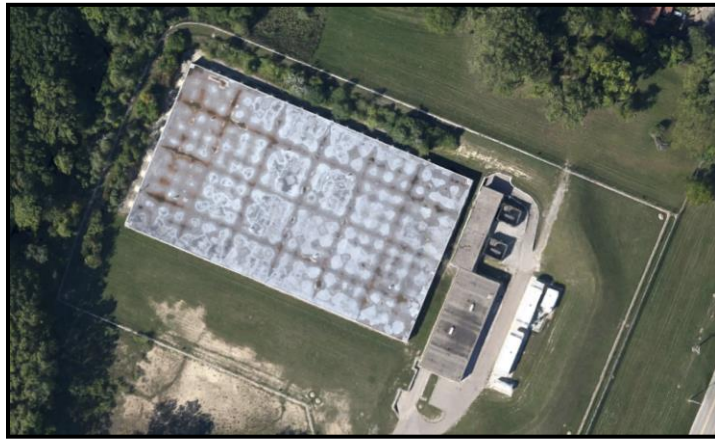
Figure VI-25. Franklin Pump Station
