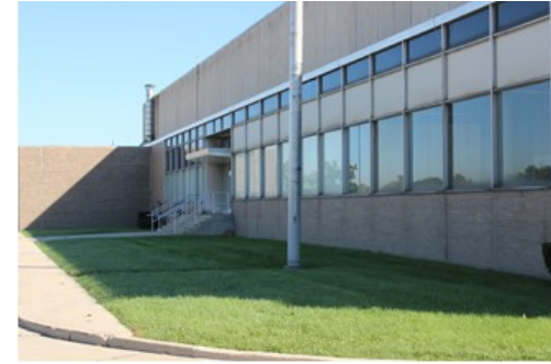
Southwest Water Treatment Plant
