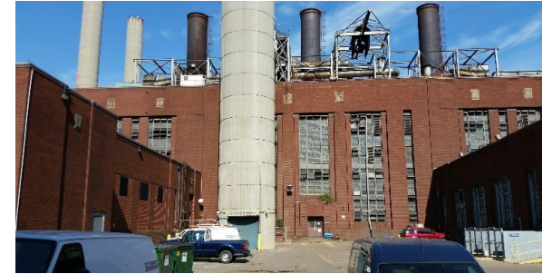
Complex – I Incinerator Building at the WRRF
