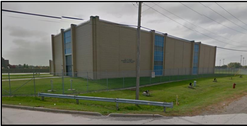
Figure VI-31. North Service Center
