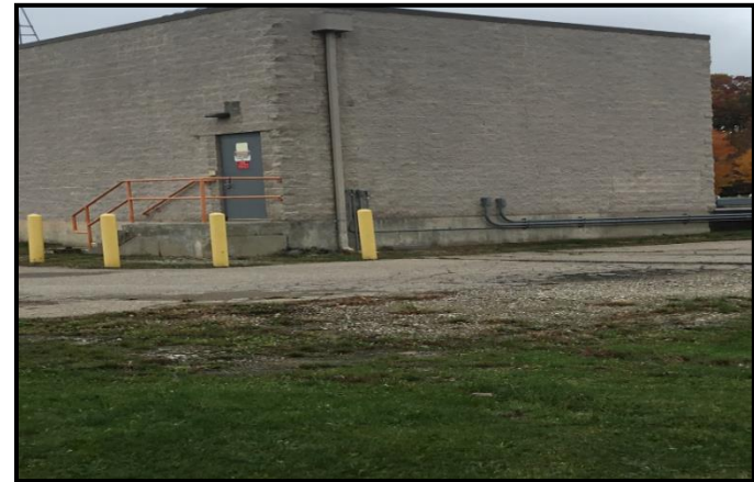
Figure VI-20. Adams Road Pump Station
