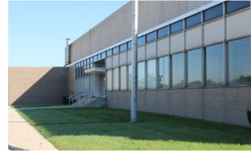
Southwest Water Treatment Plant
