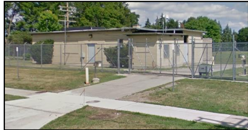
Figure VI-36. West Chicago Pump Station
