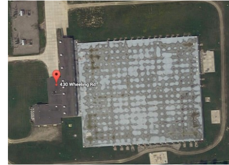
Imlay Pump Station
