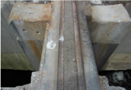
Piece of movable dam at DRO-2
