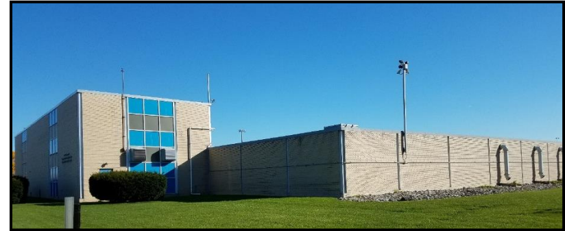
Figure VI-24. Ford Road Pump Station
