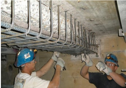
Lake Huron WTP Electrical Tunnel
