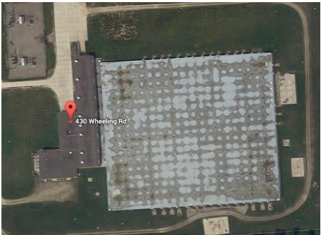
Imlay Pump Station
