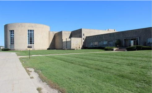
Northeast Water Treatment Plant
