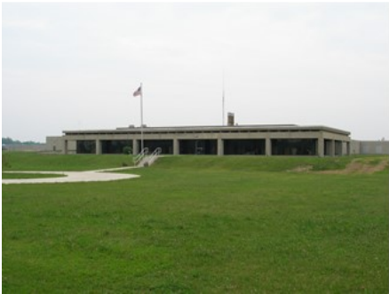
Lake Huron Water Treatment Plant
