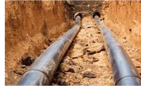
Water main installation
