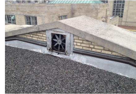
Springwells filter building
