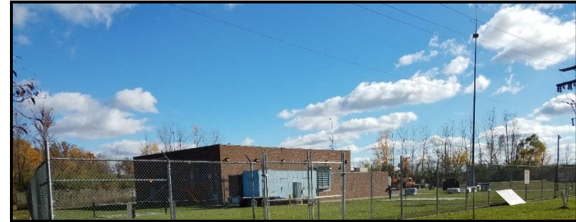
Figure VI-38. Ypsilanti Pump Station
