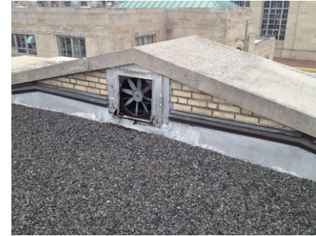
Filter Building roof
