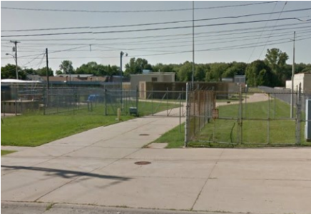
Joy Road Pumping Station
