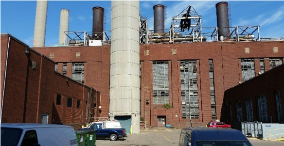
Complex – I Incinerator Building at the WRRF
