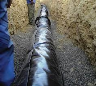
Water main being laid
