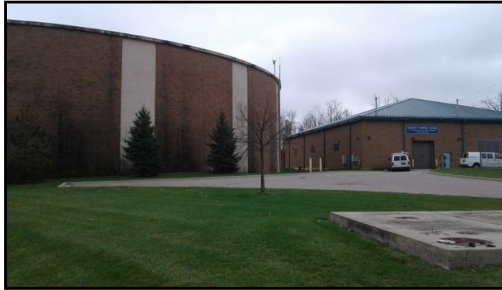
Figure VI-23. Haggerty Pump Station
