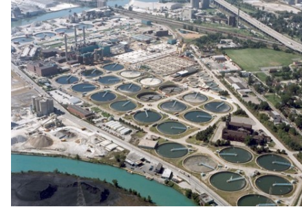
Aerial view of the WRRF
