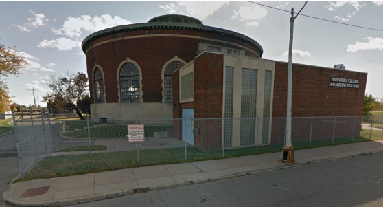
Freud Pump Station
