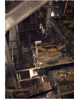
Picture from left to right Sludge Conveyer G Damaged by Fire and Conveyer B in the Complex – II Dewatering Building and Fire Damaged Conveyer H in Complex-II Incinerators Building
