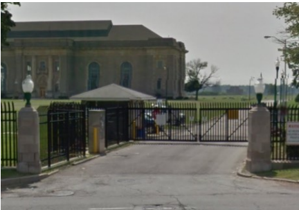
Waterworks Park WTP
