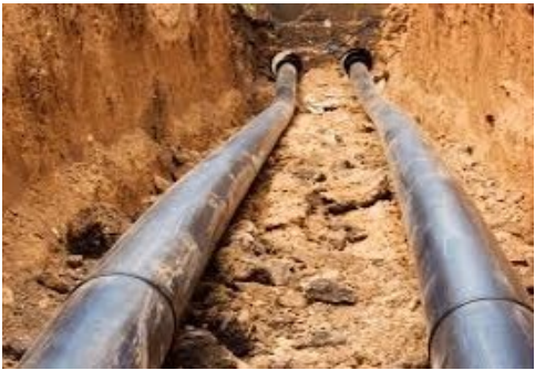
Example of pipe being laid
