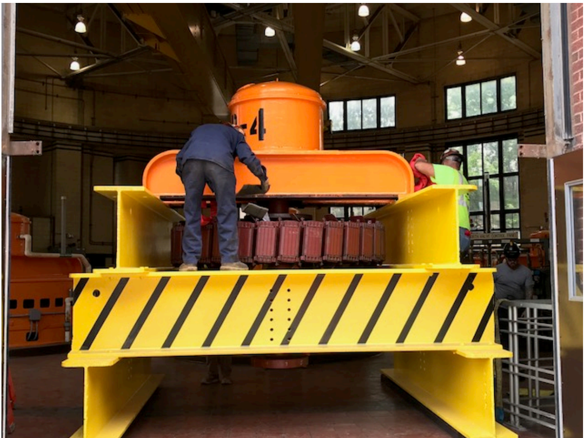
Rotating assembly for pump #4 motor ready for pick up at WRRF pump station #1
