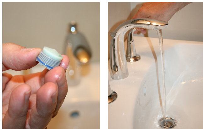
Cleaning faucet aerators monthly and running cold water to flush a faucet that hasn't been used for 6 or more hours help preserve drinking water quality in your home.
